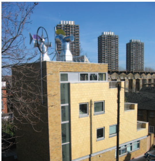
Figure 9 Wind turbine on BowZED House, 2001. Architect: Bill Dunster.
