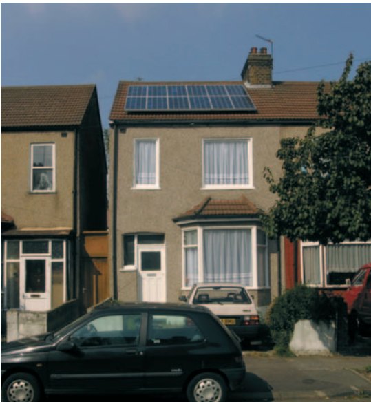
Figure 8 A typical domestic PV installation
