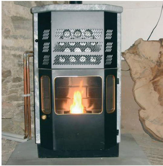
Figure 12 A wood pellet stove with a back boiler courtesy of Centre for Sustainable Energy
