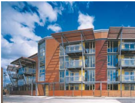
An example of permanent shading to reduce solar gains. Greenwich Millennium Village Phase 2a, Proctor & Matthew (photo: David Churchill)
